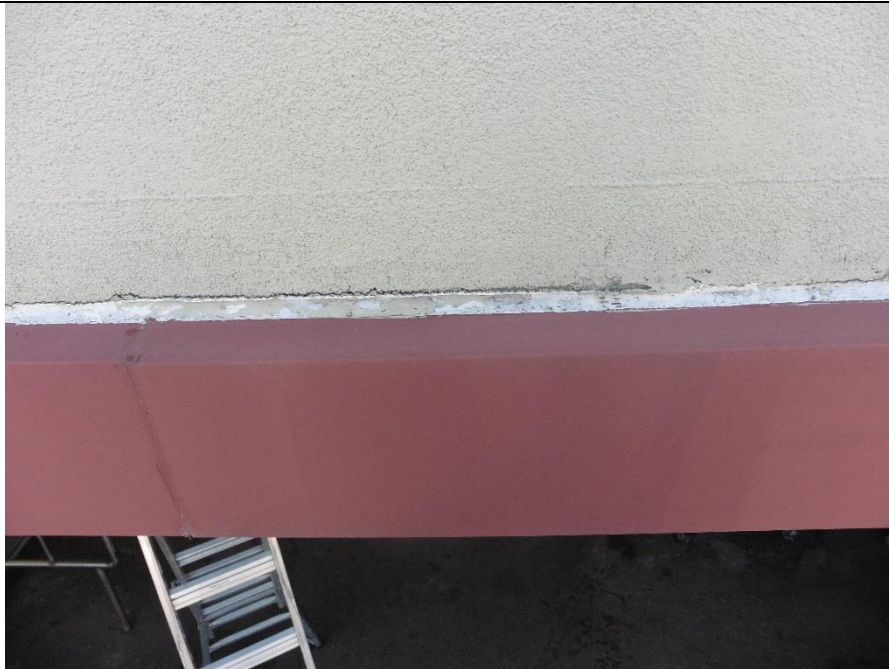
Separating caulking above the metal clad water table shelf. The EIFS siding is above.
