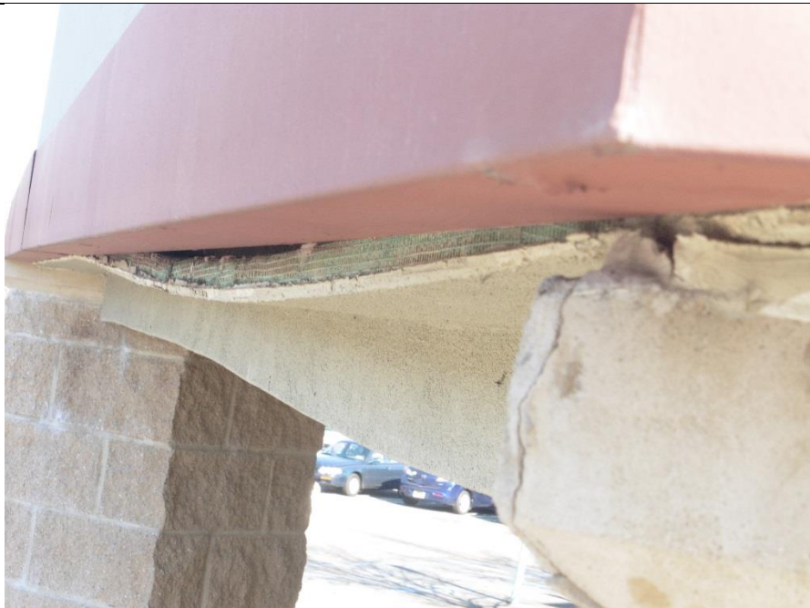
Drooping, failing EIFS at soffit on west portion of west entrance roof. This is a result of chronic seepage into soffit and lack of maintenance.
