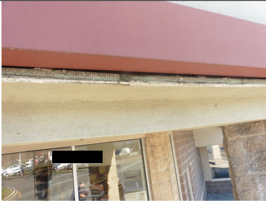
Soffit separation.
