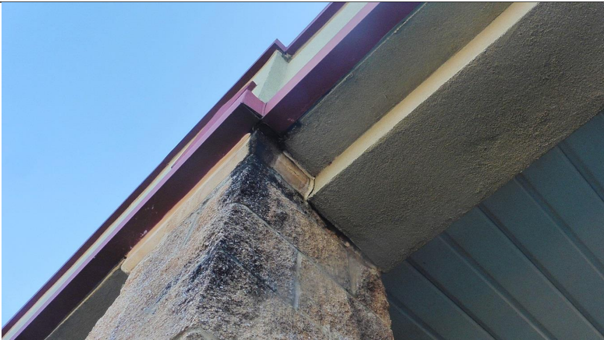
Staining at the masonry column at the west entrance from water flowing off the red metal detail known as a water table.
