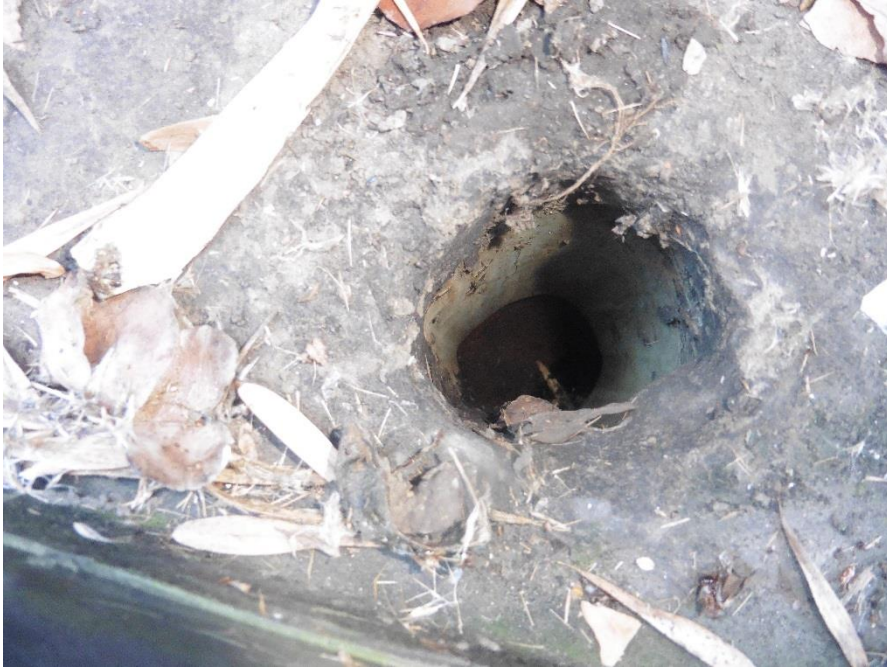
This 2 inch diameter copper drain tube is inserted into, but not sealed to, the PVC internal drain pipe.
