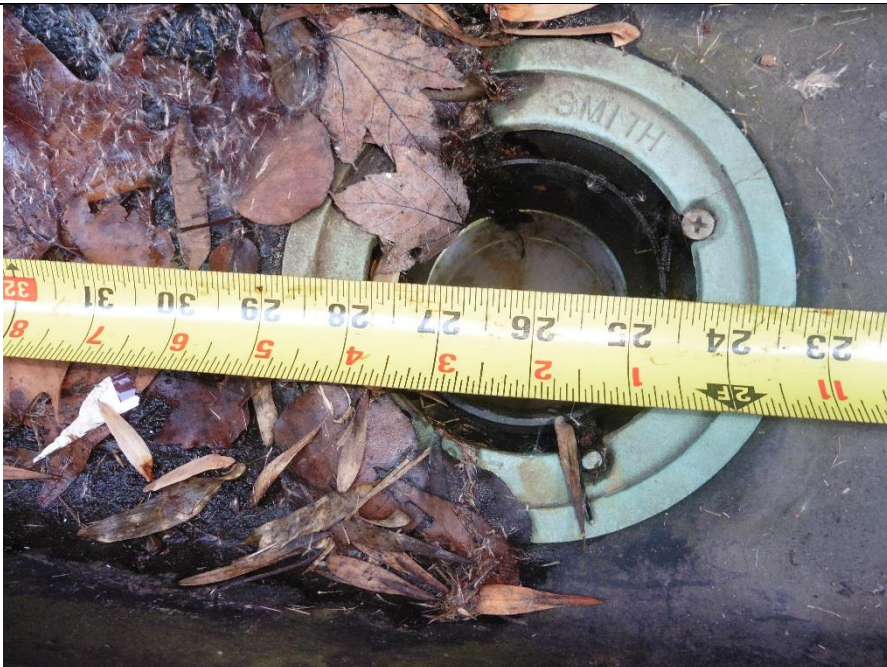
This 3 inch diameter Smith drain on the south leg of the built in gutter is sealed to the PVC pipe.
