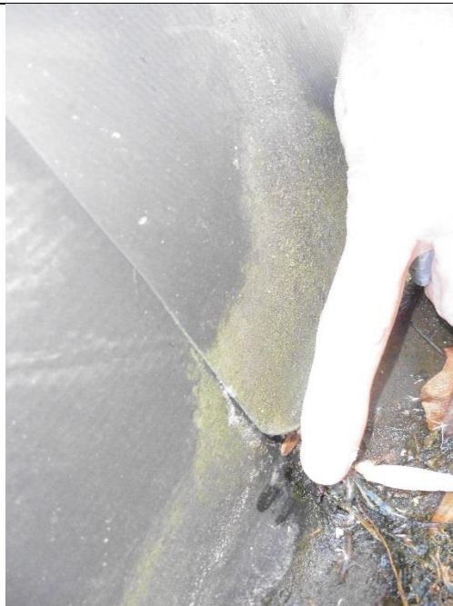
Failing seam in rubber gutter lining lacks an uncured patch required during original installation.
