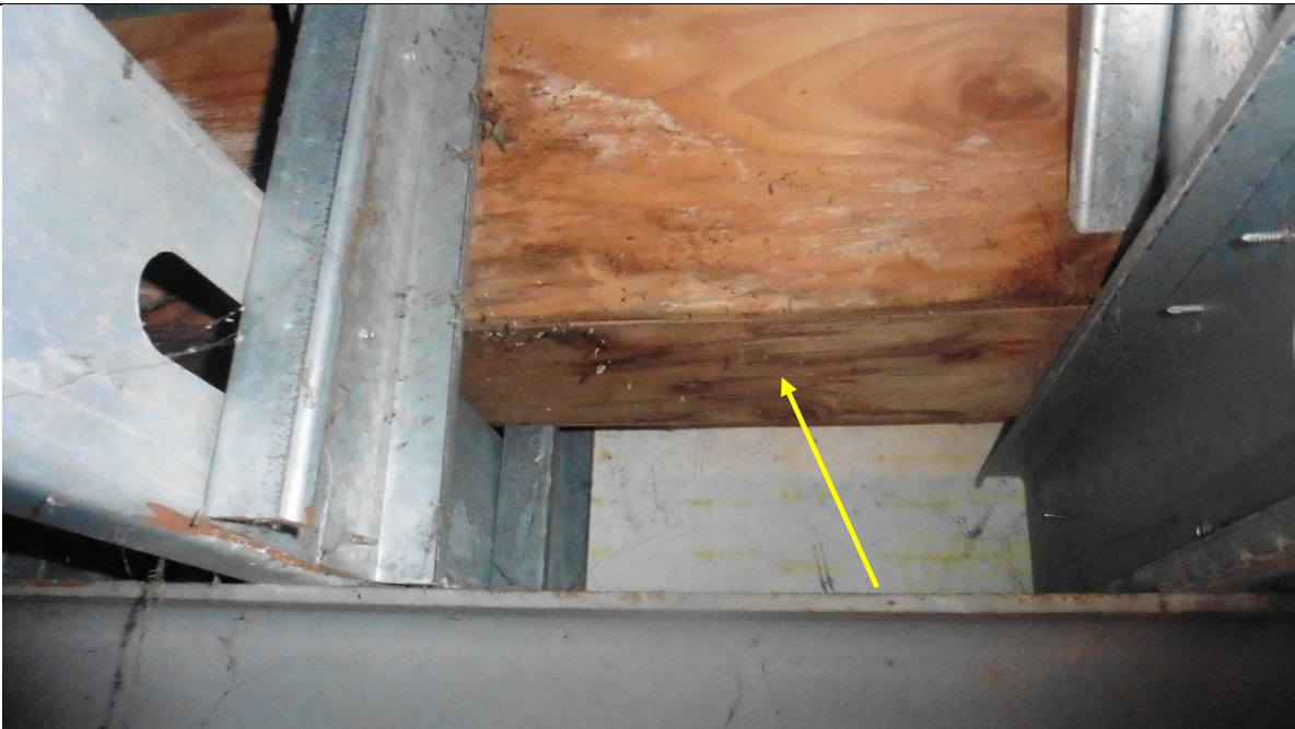
The plywood seen here is the framing of the recessed built-in gutter. Note the water staining.
