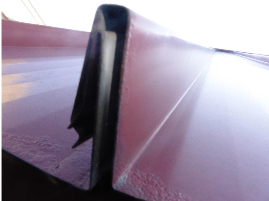
This close up photo of the standing seam roof panel shows the open seam end is susceptible to wind driven rain.
