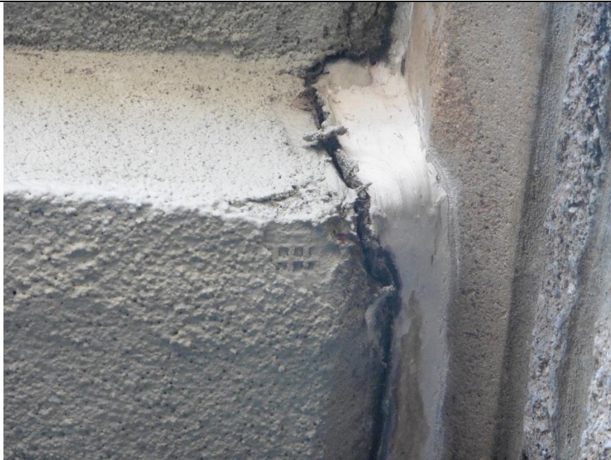
Deterioration and separation in the EIFS where it was used on a horizontal surface with no flashings.
