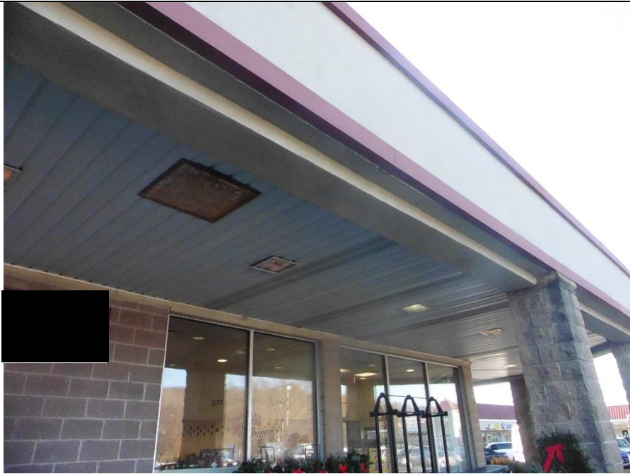
Access hatch for soffit.
