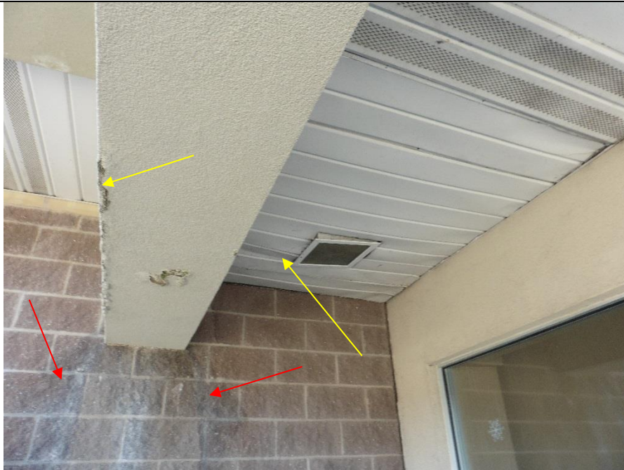
Soffit damage (yellow) and efflorescence (red, mineral stains) in the masonry from chronic seepage from the gutter above.
