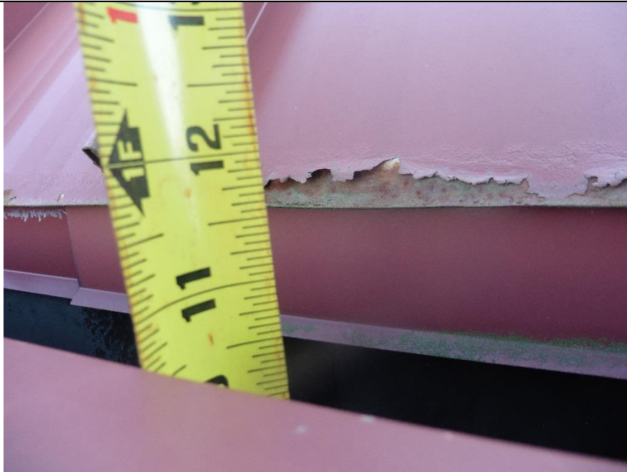
The gutter is approximately 10.75 inches deep at the front.
