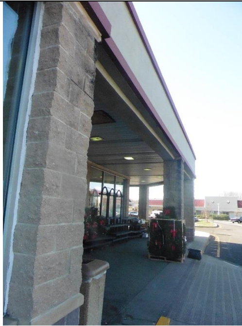
The drains for the gutter run inside the masonry columns, an almost perpetually shaded area in the winter.
