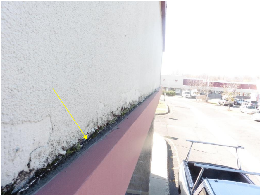
EIFS deterioration.
