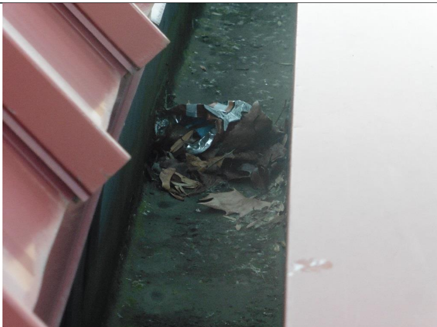
This accumulated debris is at a roof drain near the hatch.
