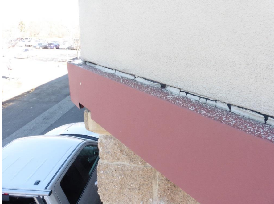
Failure of the caulking joint at the corner jog in the front facade.
