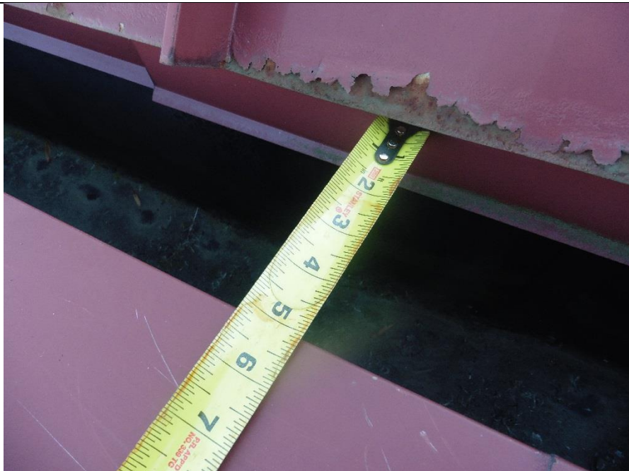
The built in gutter is 5 inches wide.
