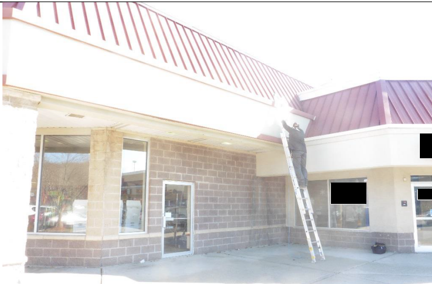
Soffit damage (yellow) and efflorescence (red, mineral stains) in the masonry from chronic seepage from the gutter above.
