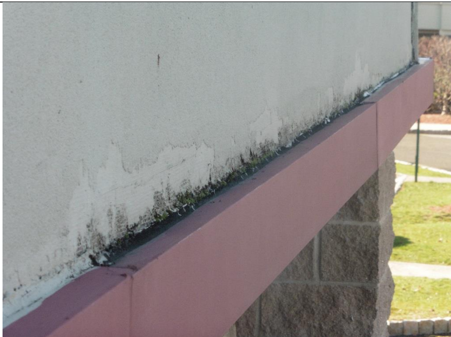
Deterioration of the EIFS is from water that accumulates on the water table band. This same water reaches the sidewalk.
