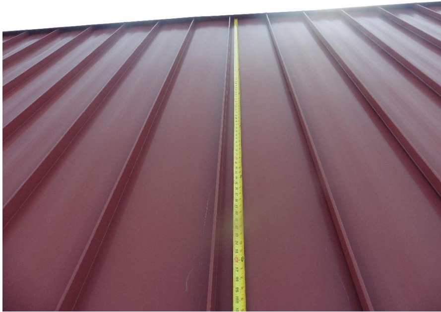
The mansard roof is constructed of standing seam, snap-lock, 24 gage steel panels, approximately 11 feet long.
