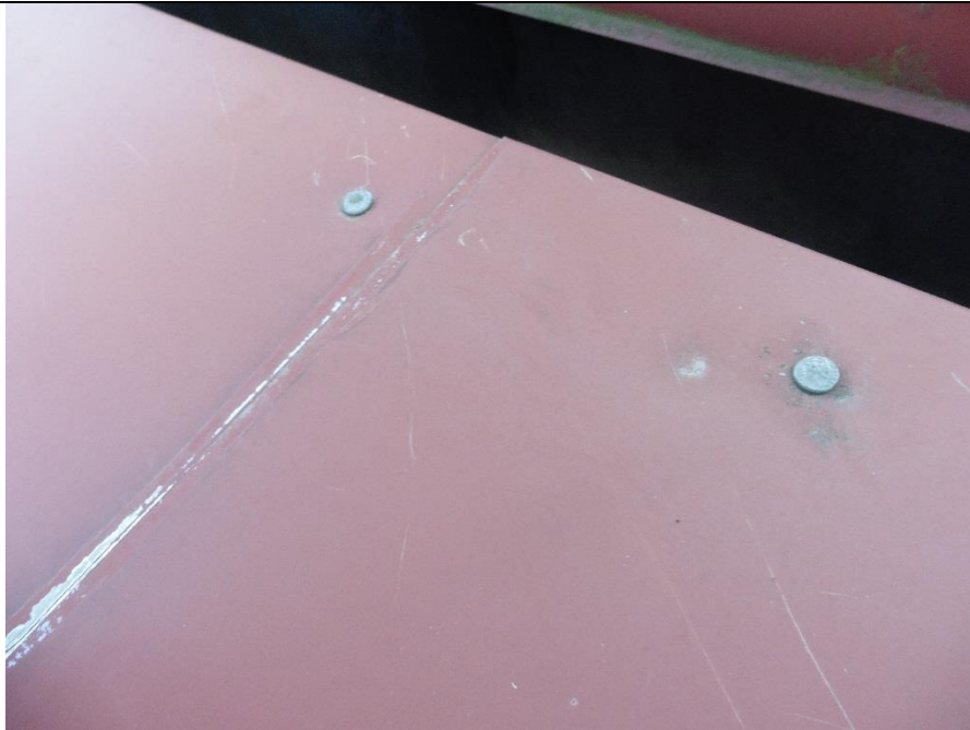
Face nails in the coping are not caulked.
