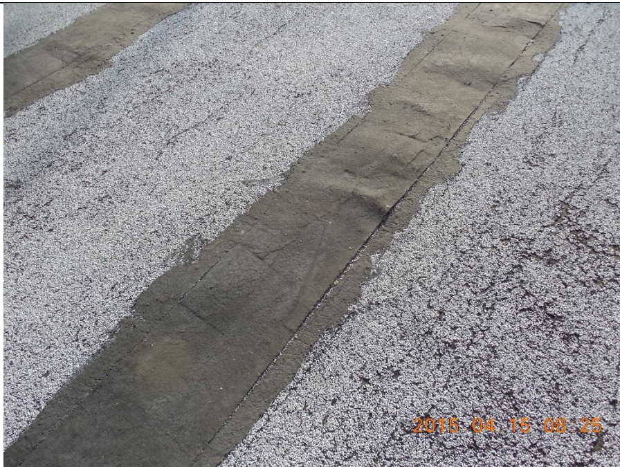
Repairs over seams are failing. Membrane is cracked and split.
