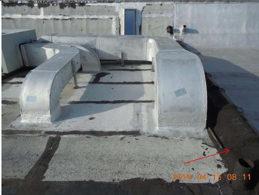
No proper flashing at duct penetrations. Modified bitumen membrane has been installed over parapet wall along northeast adjoining wall (red).
