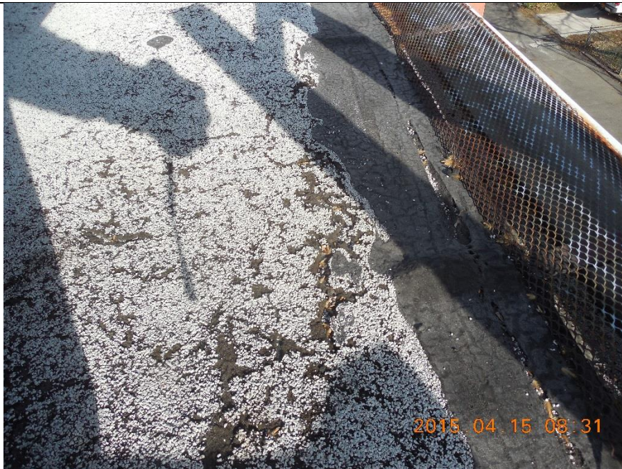
Worn out roof above gutter.
