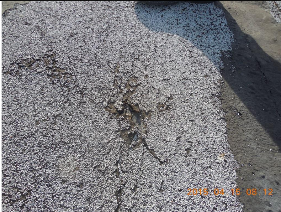
Roof membrane has worn through in numerous locations.
