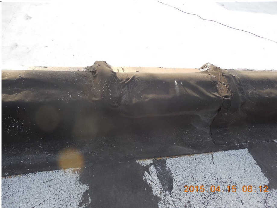
Modified bitumen membrane on parapet wall. Water can seep under roof system where modified bitumen overlaps granular surface roofing at perimeter of roof.
