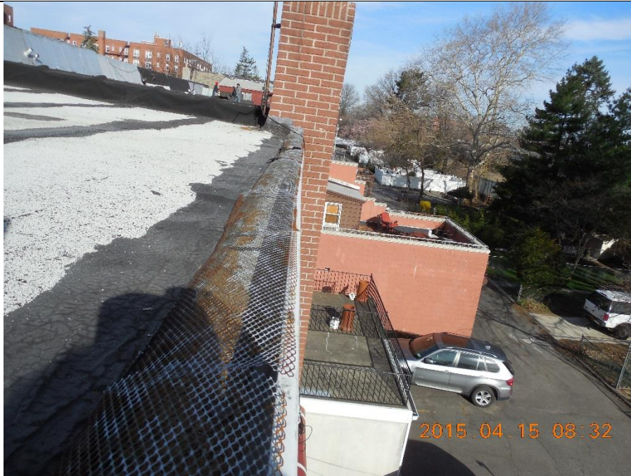
Overview of back edge of roof with elevated gutter.
