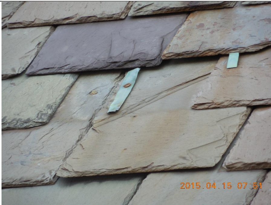
Missing slate on front upper roof. Copper strap failed from years of exposure.
