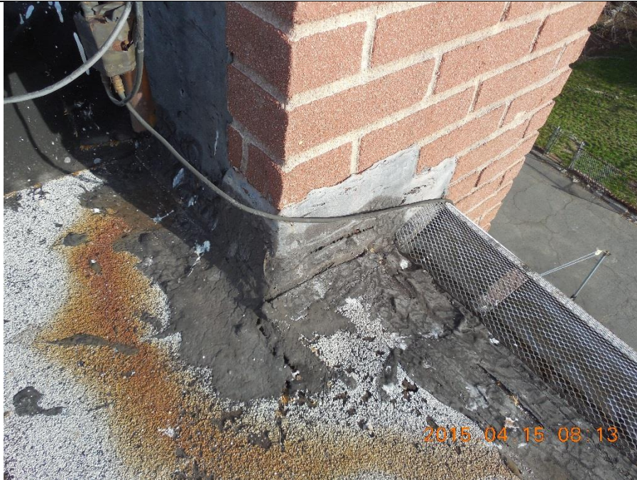
No proper flashing at chimney. Failed flashing and membrane at base of chimney.
