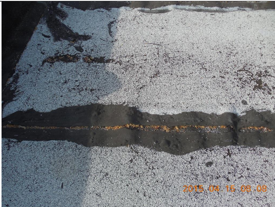
Failed seams and worn out membrane.
