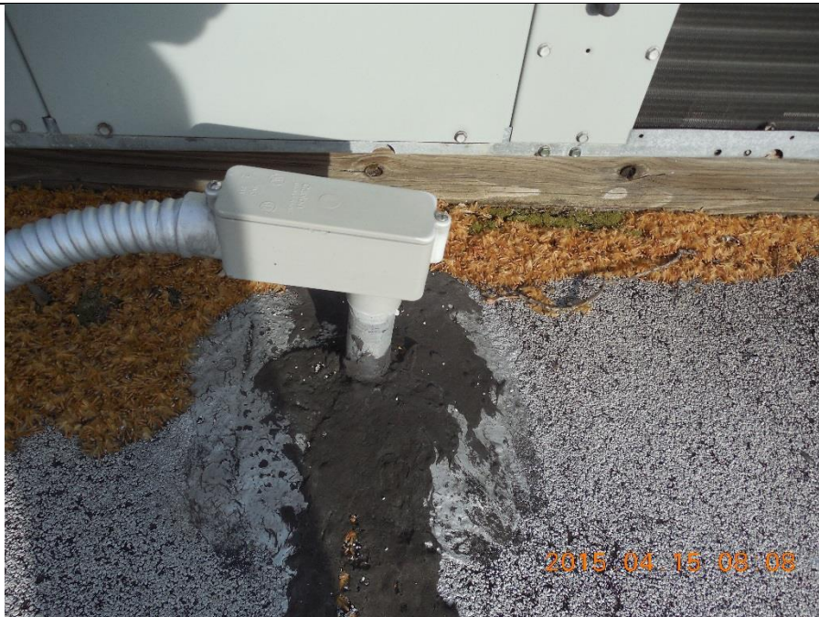
No proper flashing at conduit penetrations.
