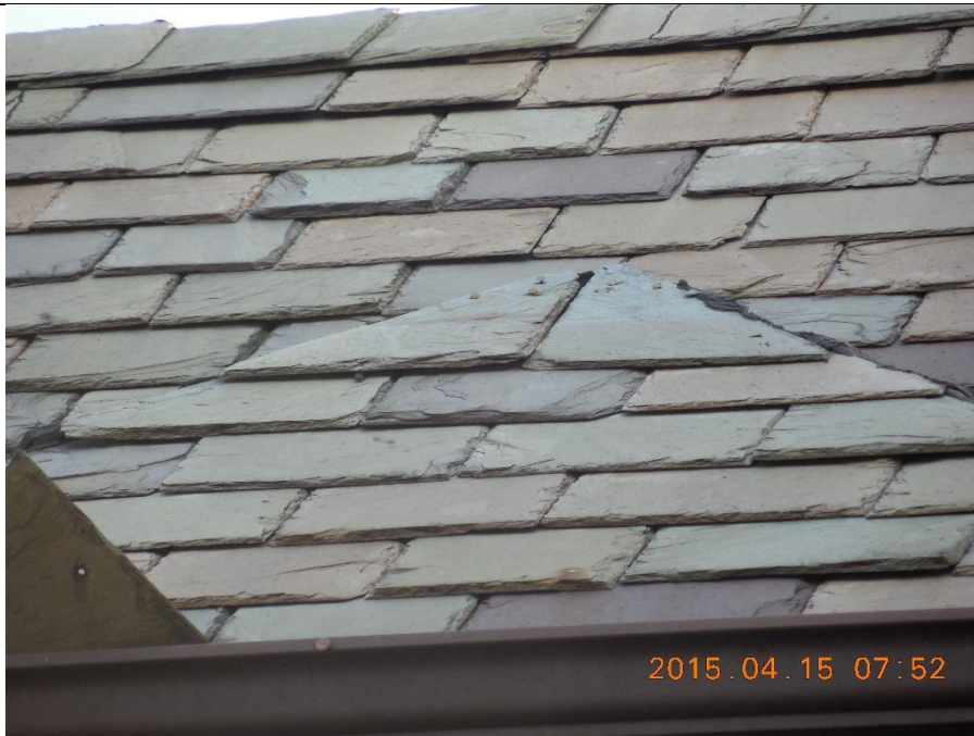
Dislodged slate from top of doorway roof. Slate is in gutter (bottom left of photo).
